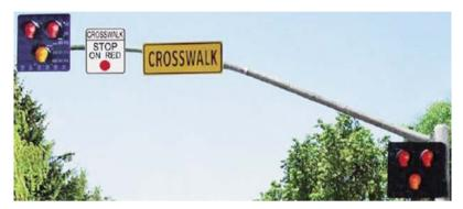
The High intensity Activated crossWalK (HAWK) pedestrian crossing beacon consists of two red lenses positioned over a single yellow lens. The traffic lights are located both on a mast arm over the roadway and on the roadside
